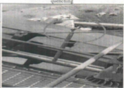
Sprinkler installed on Ash Conveying belt for quenching
