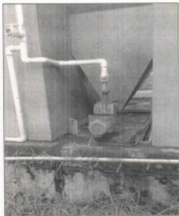
ANNEXURE 5 - SLUDGE RECIRCULATION PUMP
